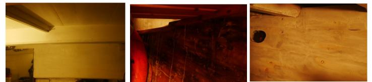
Middle is conditions across under the bed and roof as well, and across right is 2 layers ground, and left is Groundpaint 3 times, fill in holes Oilpaint 1 Sanding and 2 layers oilpaint to make
